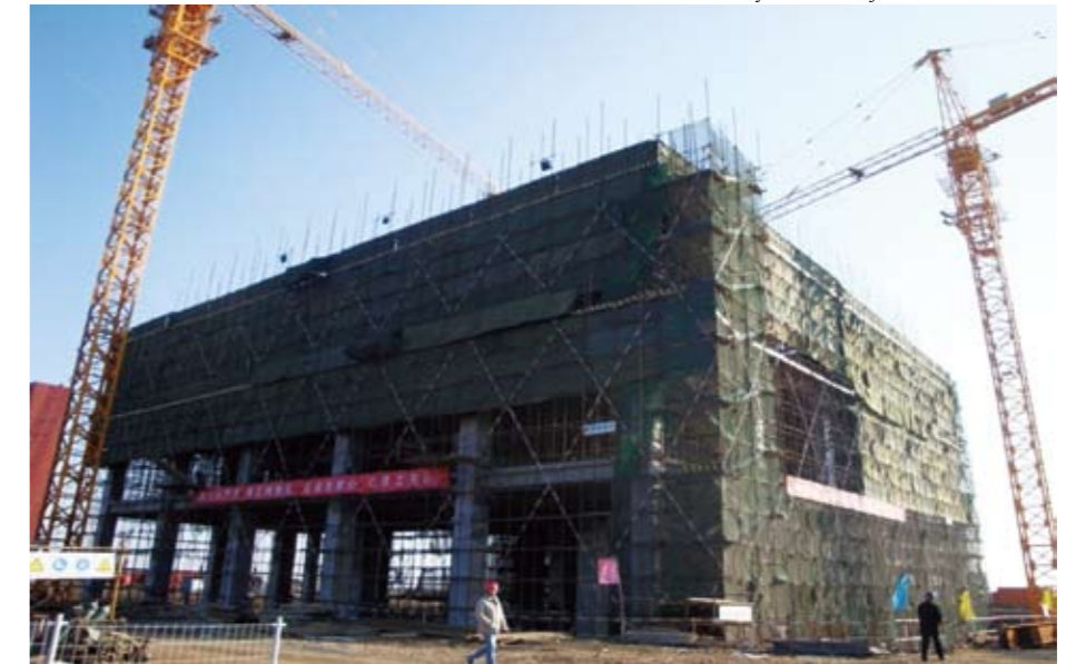
● Coal Gasification System at Tianjin IGCC Power Plant
