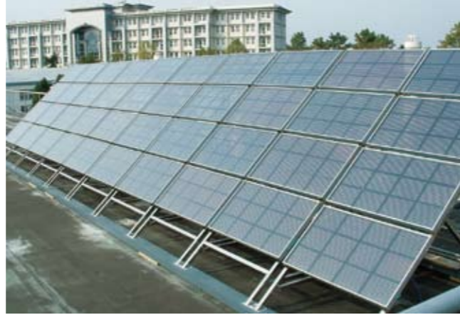
● 500W Dye-Sensitized Solar Cells in Hefei, Anhui Province
