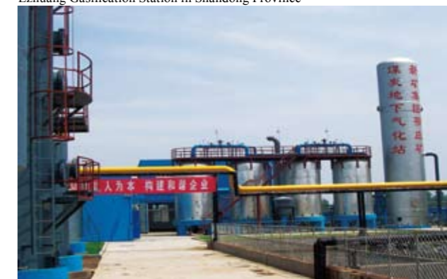
● Oxygen Making and Coal Gas Purification System at Ezhuang Gasification Station in Shandong Province
