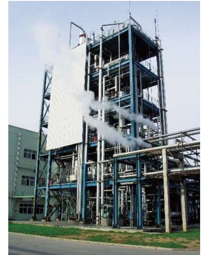
• Low Temperature Slurry Bed 5,000 Ton F-T Installation at Yanzhou Coal Mining Group in Shandong Province
